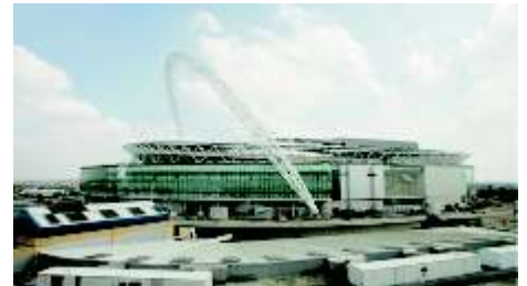
An external view of Wembley Stadium, July 2006
